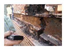
Deteriorated steel beam found hidden in a masonry wall. Brick and mortar replacement studies.
