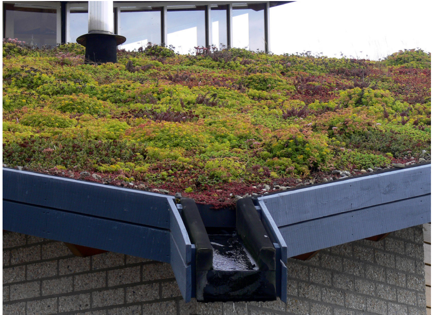
Green roof in Culemborg, The Netherlands. Image Credit: Lamiot. ▶
