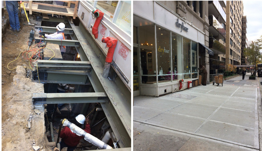
Sidewalk vault repair before and after. ▶
